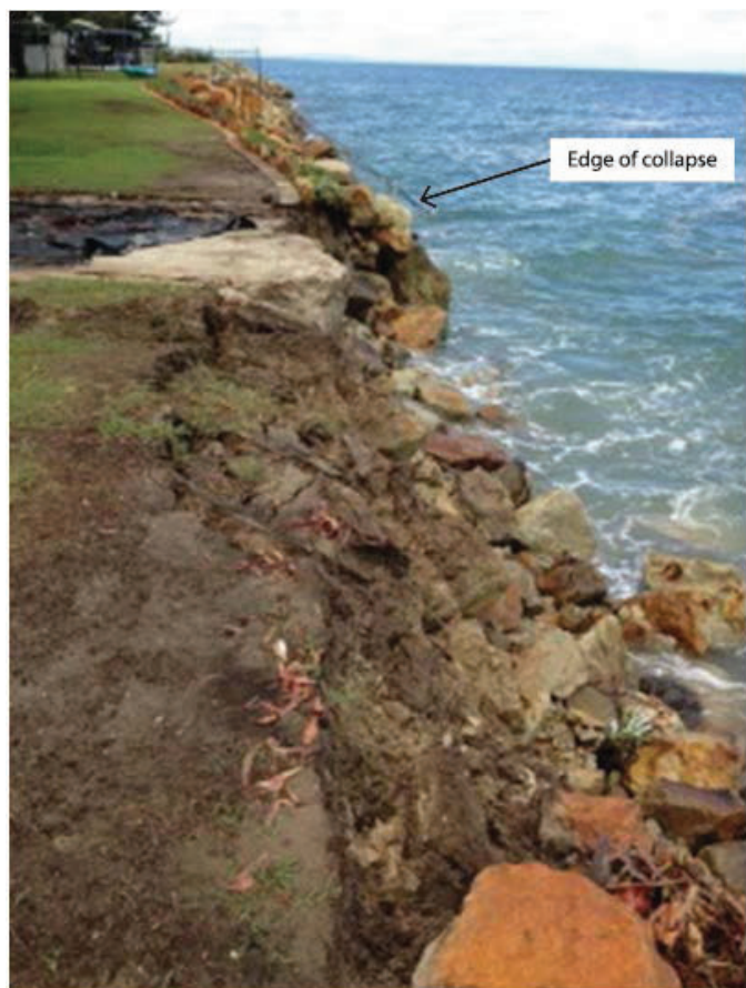
Fig. 7: A 22m wide seawall slump at Amity Point occurred 7.12.2014.
