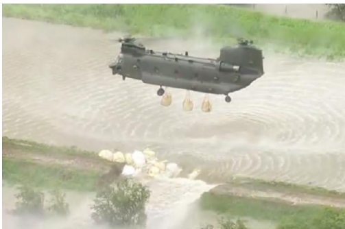
Figure 5: Deployment of Chinook helicopter in dyke breach Wainfleet, 2019
