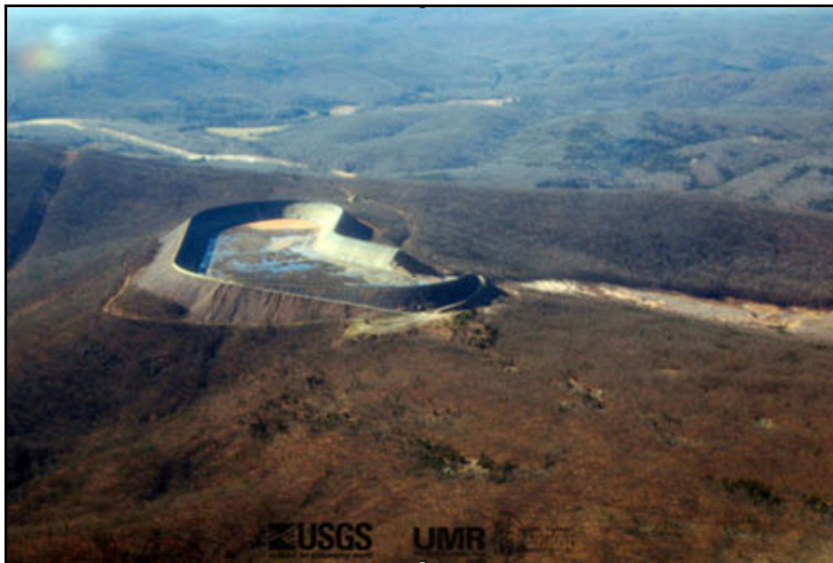
Figure 4.1. Aerial photo of the Taum Sauk Upper Reservoir, just after breach in December 2005.
