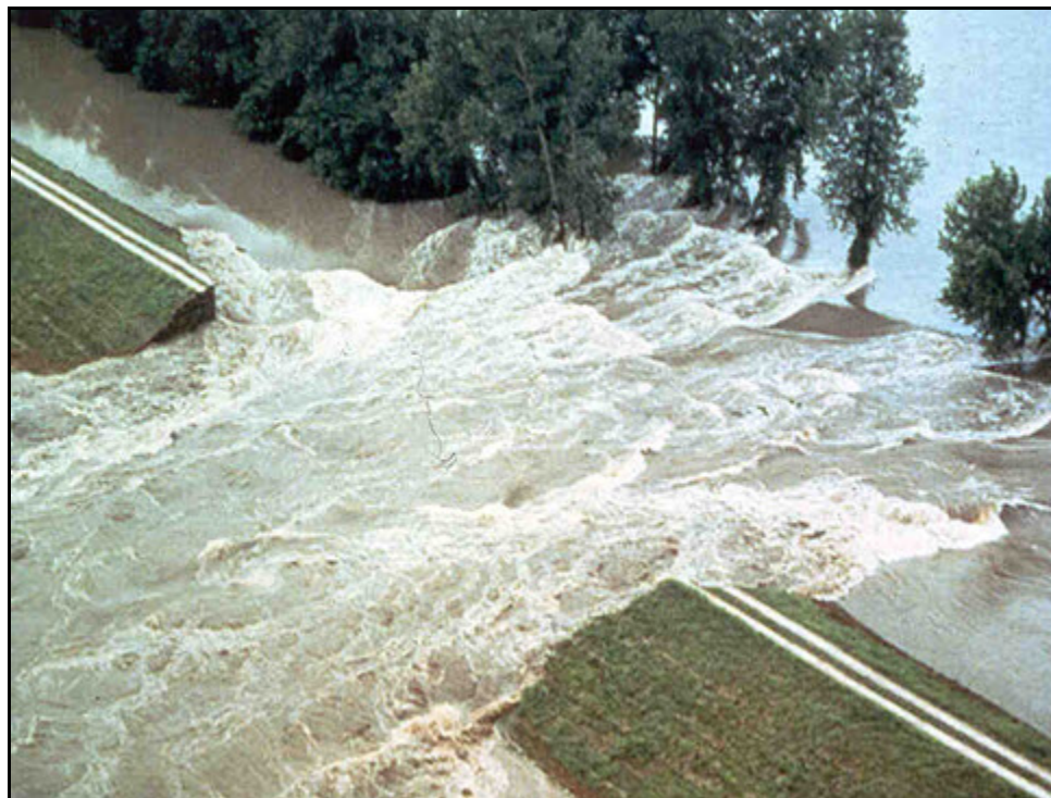
Figure 3.12. Kaskaskia River levee breach at location of sand boil.
