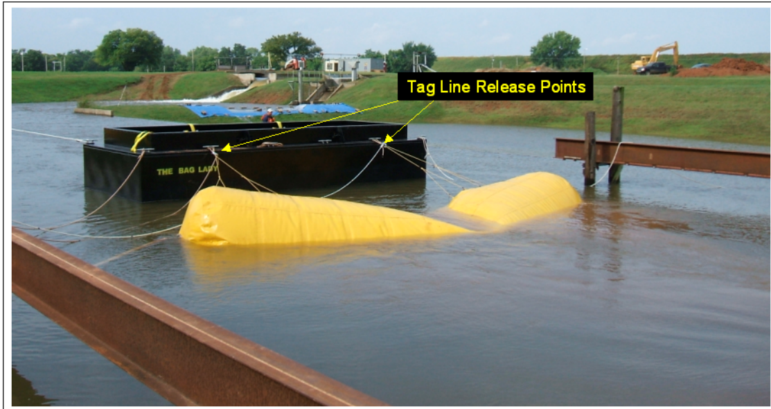
Figure 5.3.2.1: Barge-Deployed Tube Configuration
