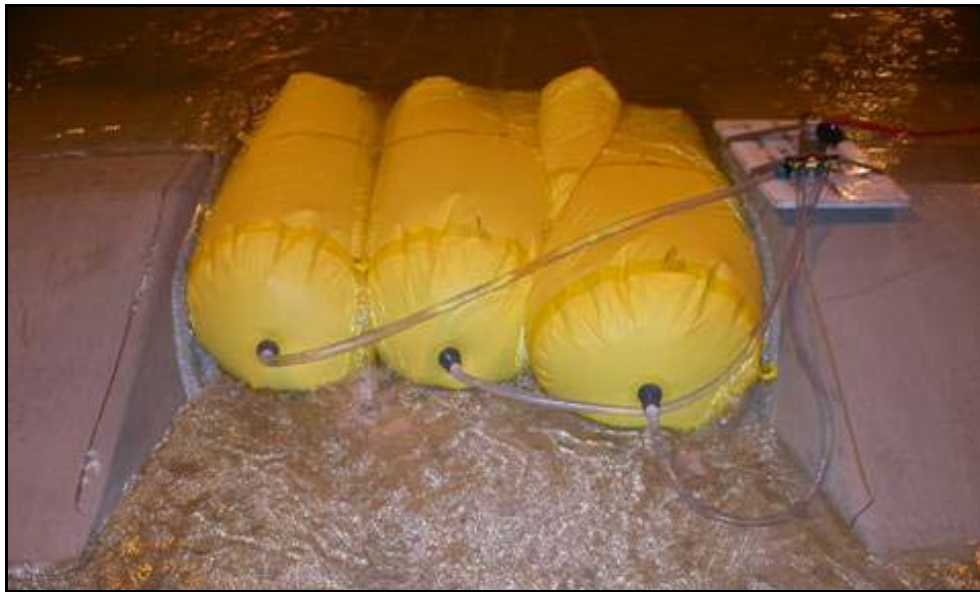
Figure 11. 30-ft-diam bags placed side-by-side to span the breach, looking upstream into the breach
