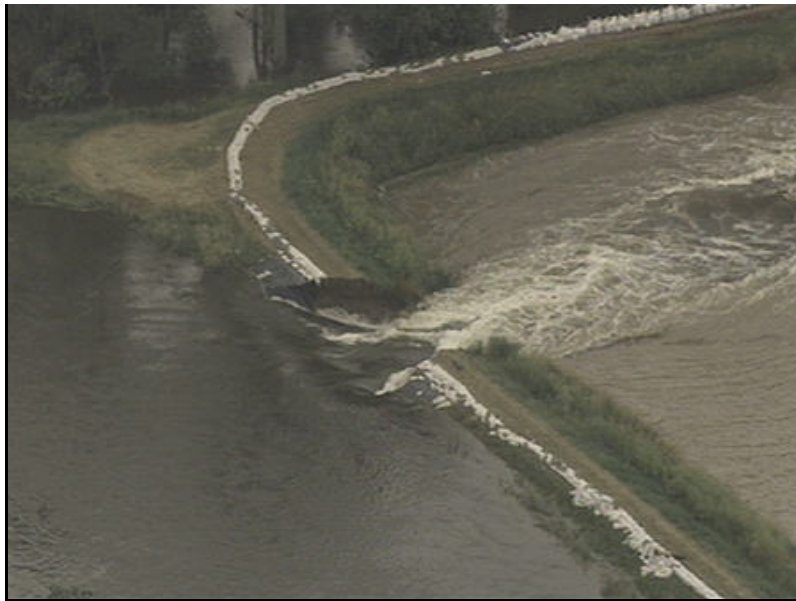
Figure 3.1. Failure of the Pin Oak levee in Midwest. Note sand bags atop levee used to fight rising water levels.
