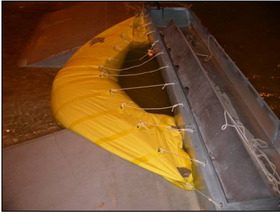
Figure 8. Bag extending into the breach while attached to the barge.
