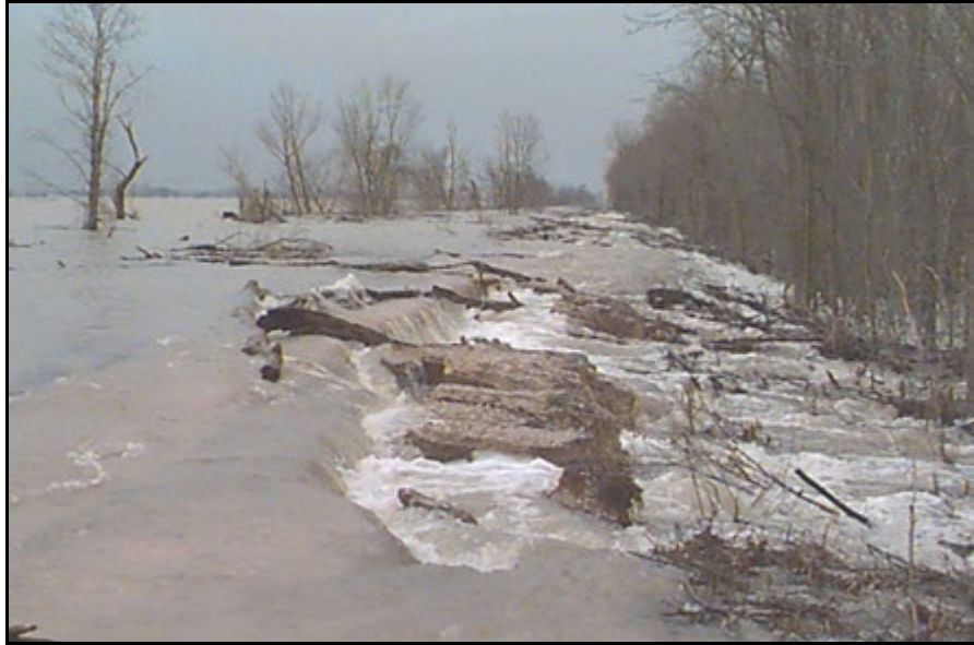
Figure 3.9. Overtopping of a levee over a wide area with a potential breach growing in foreground.
