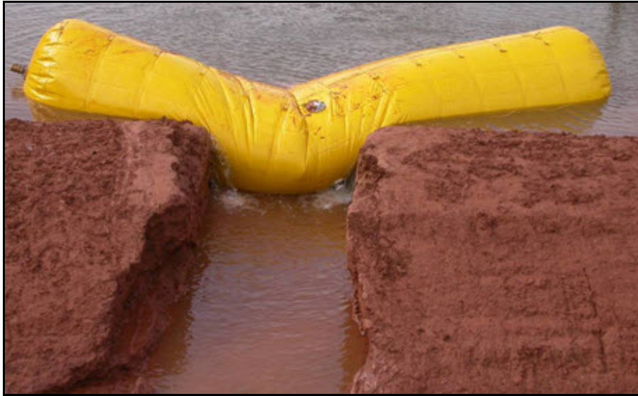
Figure 7.6. Sample deployment of deep-breach closure system, with a small residual flow still persisting along the upper edges of the breach opening.
