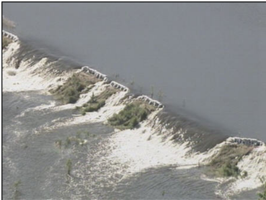
Figure 3.10. Overtopping of the Foley levee in the Midwest.
