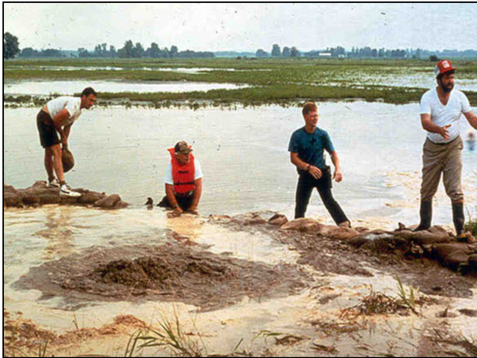
Figure 3.11. Sand bag levee around sand boil on Kaskaskia River. Notice that one guy in this picture, who appears to be the oldest guy, has doubts about whether this is going to work because he is wearing a life vest.
