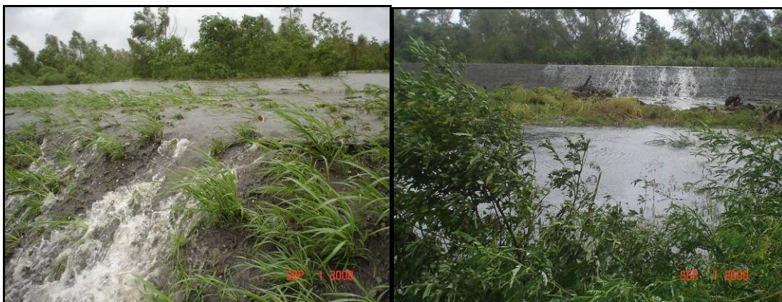
Figure 7.5. Two photos from overtopping in Braithwaite, Louisiana during Hurricane Gustav. The left-hand panel shows a close-up of flow over a low area along the levee crest, while the right-hand panel shows a wider perspective of this flow.
