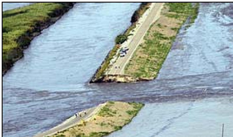
Figure 3.3. Upper Jones Tract levee Breach in the Sacramento-San Joaquin River Delta.
