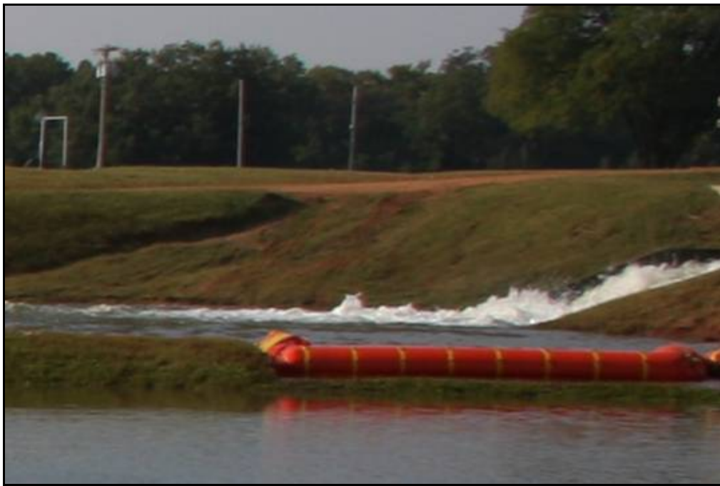
Figure 7.3. Demonstration of shallow, wide breach closure system at ARS facility in Stillwater.
