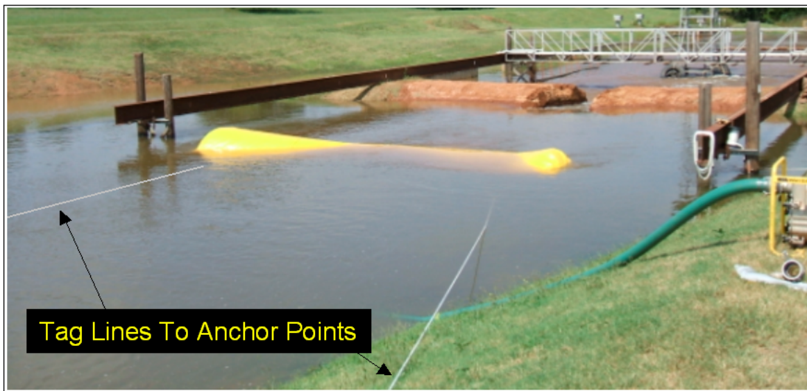
Figure 5.3.1.1 Tube Filled, Staged for Deployment
