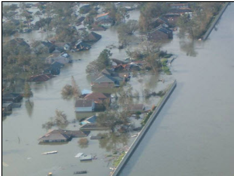
Figure 3.4. Floodwall failure on 17th Street Canal from Hurricane Katrina in New Orleans.
