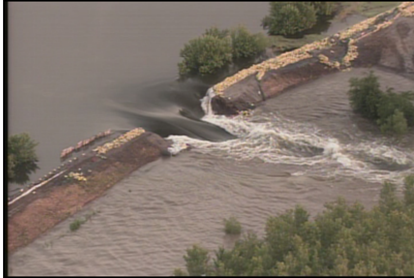
Figure 3.2. Failure of the Elm Point levee in Midwest.
