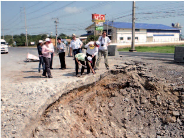
Figure 3.5 Measuring the breach in the Manorom dyke near Chainat (location km 2 +650)
