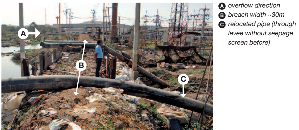
Figure 3.12 Breach at Rojana Industrial Estate (location 2) from canal side
