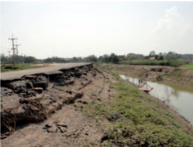
Figure 3.2 Erosion on the inner slope of the dyke and the asphalt road of a dyke near the Klong Ta Nueng floodgate
