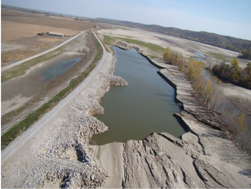
c: Emergency rock placement after the flood receded
