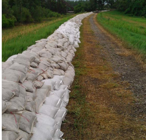
g. Sandbags used to raise levee crest to prevent overtopping
