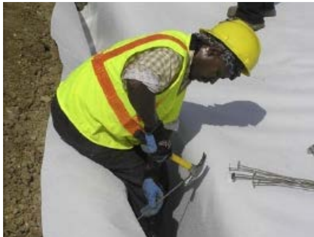
c: Anchoring HDPE in Anchor Trench
