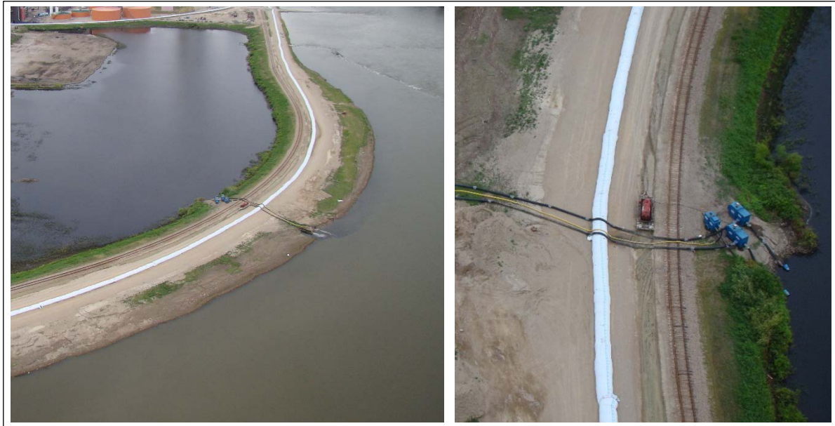
Figure K-31. Deployment of Water Filled Bladder Flood Barrier for Levee Raise.
