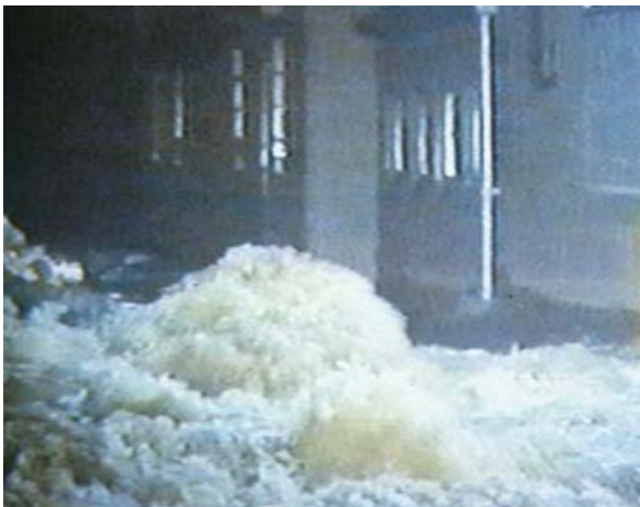
e: Very Large, Very High Activity Concentrated Leak under floodwall
