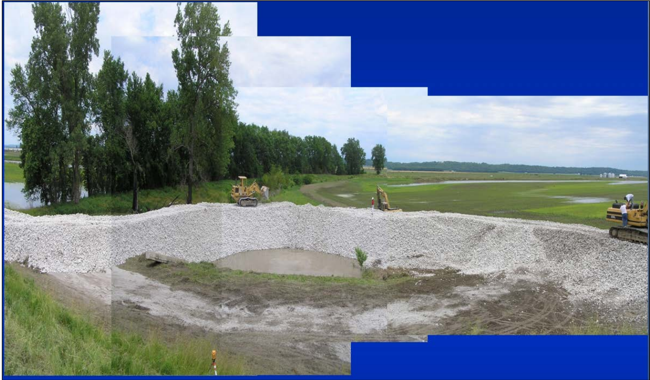
Figure K-23. Full Height U-Shaped Flood Barrier Constructed Landside to Prevent Flood Waters from Entering the Leveed Area through a Drainage Structure with a Failed Riverside Closure Structure.
