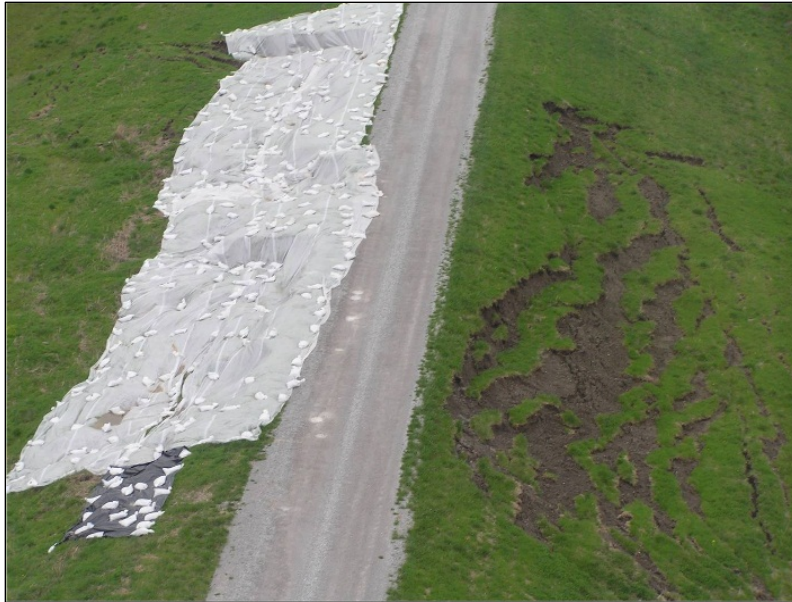
Figure K-19. Poly Installed on Riverside Slope to Reduce Through-Seepage in Area of Slope Distress.
