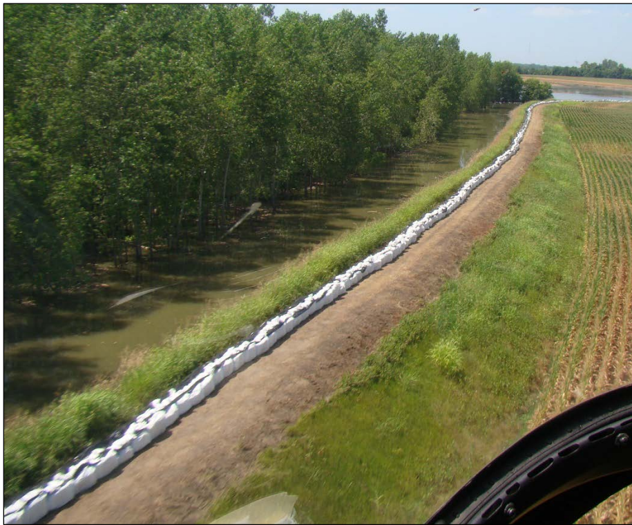
Figure K-33. Deployment of Large Sand Bag Flood Barrier to Raise Levee.
