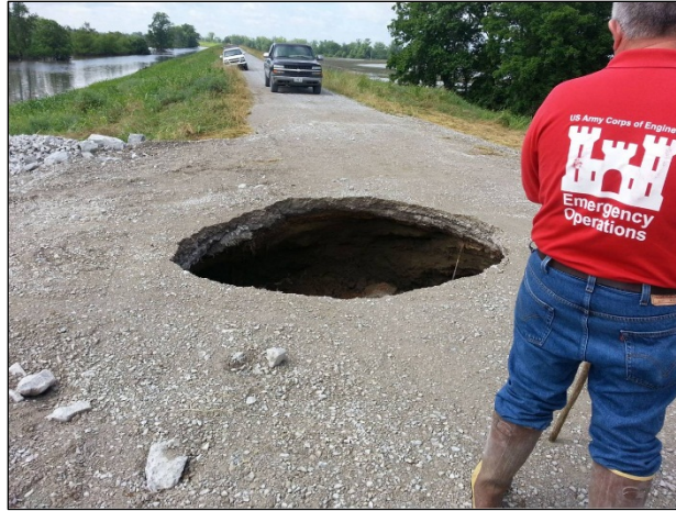
Figure K-9. Sinkhole in Levee over Gravity-fed Drain Pipe.
