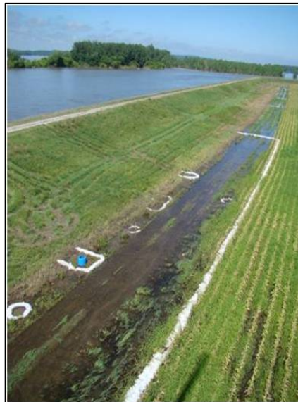
Figure K-15. Multiple Sandbag Rings along Levee Toe with Larger Ring Around Entire Area Constructed Later.
