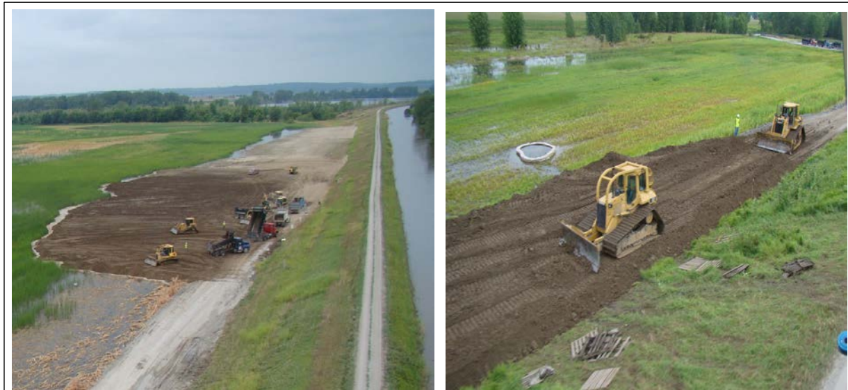
Figure K-17. Construction of an Emergency Underseepage Berm.
