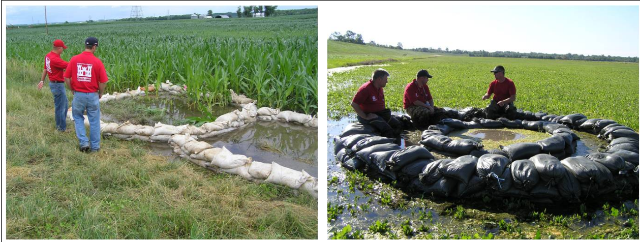
Figure K-13. Multiple Sand Bag Rings.
