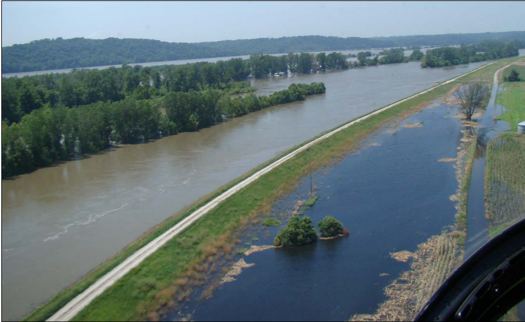
Figure K-8. Turbulent Flow Observed Adjacent to Levee that Caused Significant Riverside Scour. Note Trees Concentrating Flow Parallel to Levee.
