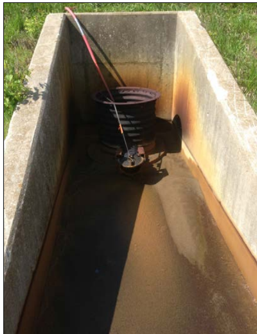
Figure K-6. Sanding Relief Well.
