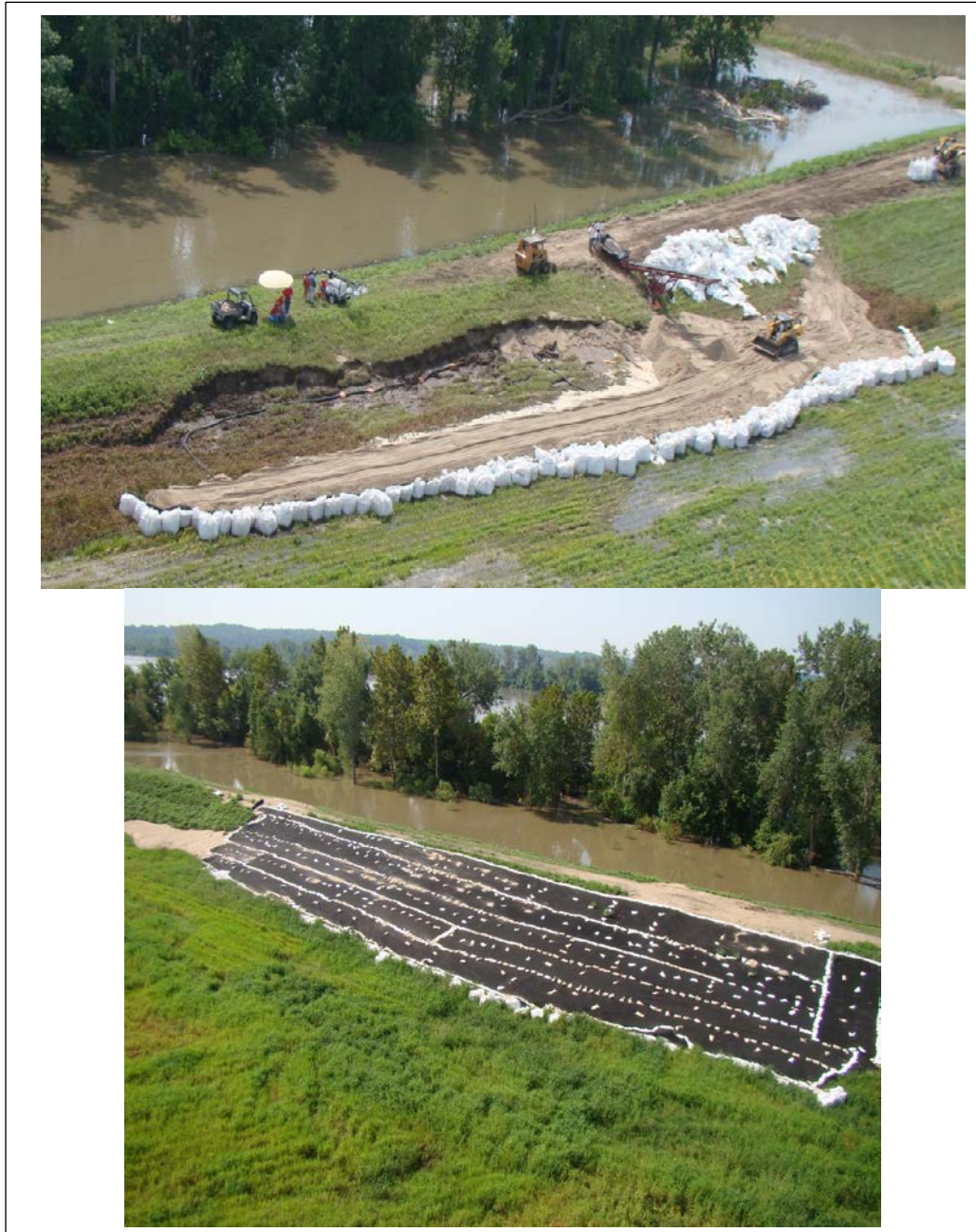
Figure K-20. Emergency Stability Berm, Under Construction and Completed. Large Sand Bags Were Used For a Toe Buttress to Reduce the Amount of Material Needed.
