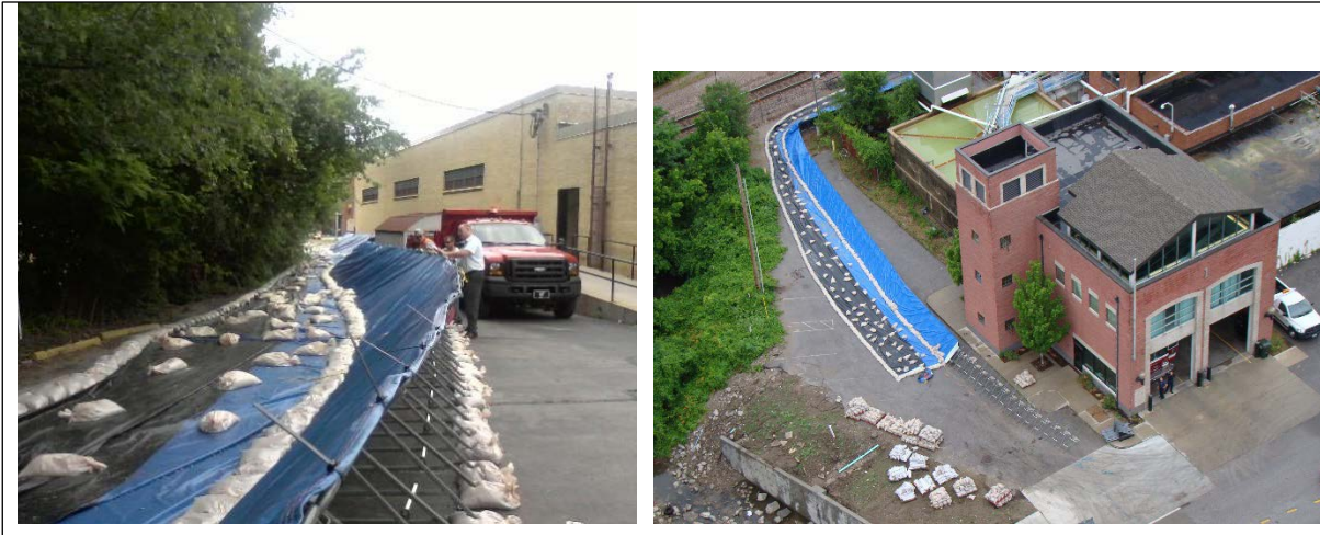
Figure K-32. Deployment of Frame Supported Waterproof Membrane Flood Barrier.
