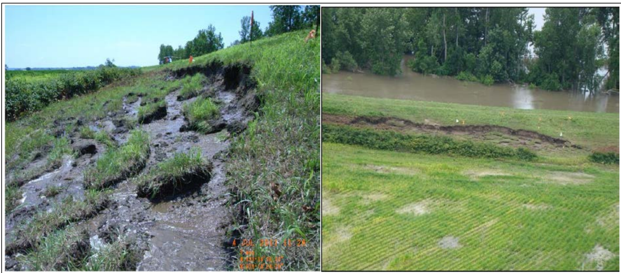
Figure K-1. Landside Slope Instability.
