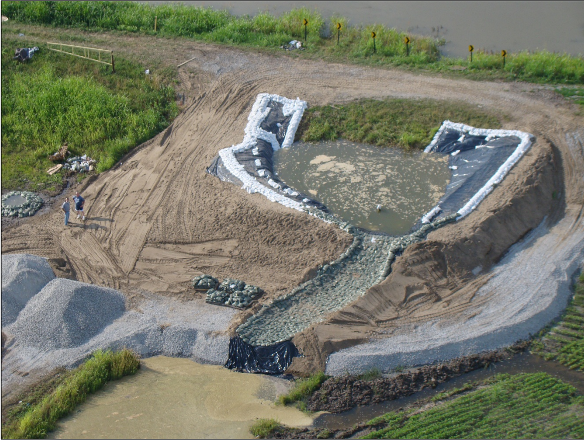
Figure K-22. Full Height Flood Barrier Constructed to Prevent Flood Waters from Entering the Leveed Area through a Drainage Structure with a Failed Flapgate.
