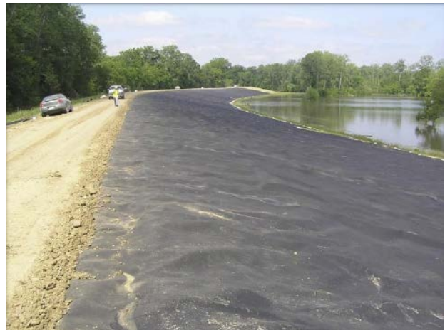
d: Completed HDPE Installation
