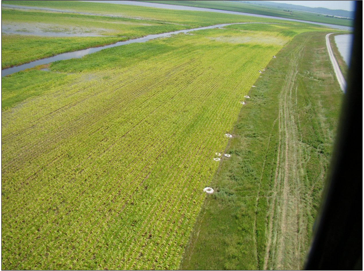
Figure K-5. Sand Boils Concentrated at Toe of Underseepage Berm.
