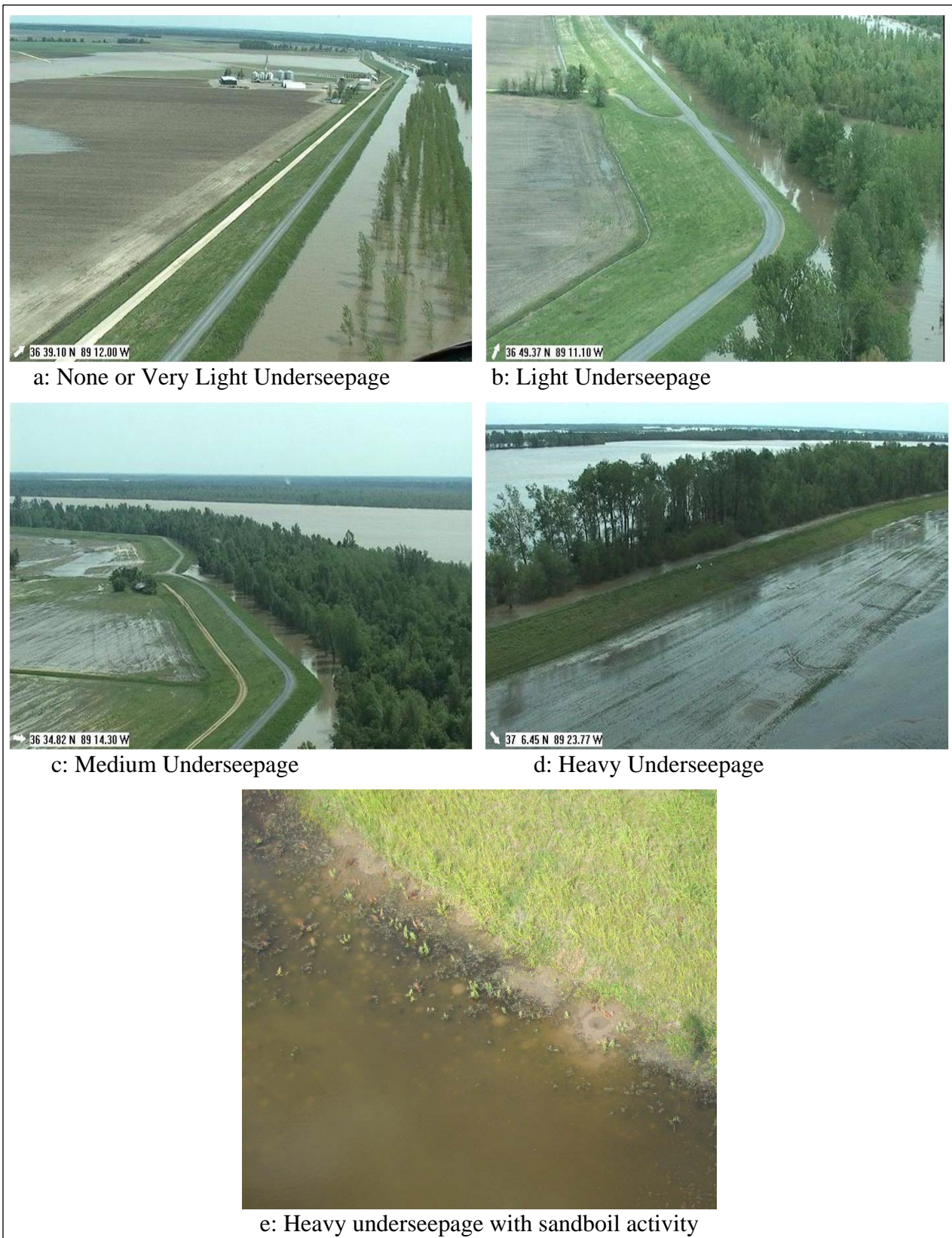
Figure K-2. Examples of Underseepage Magnitude.
