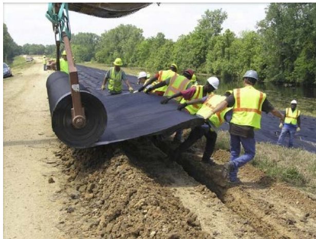
a: Deploying HDPE on Landside Slope
