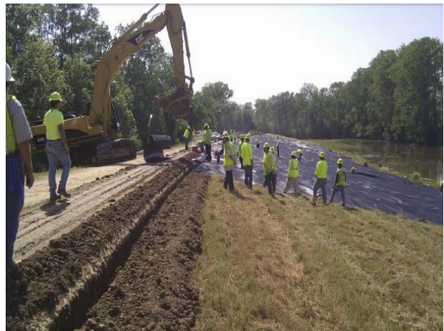
b: Deploying HDPE on Landside Slope
