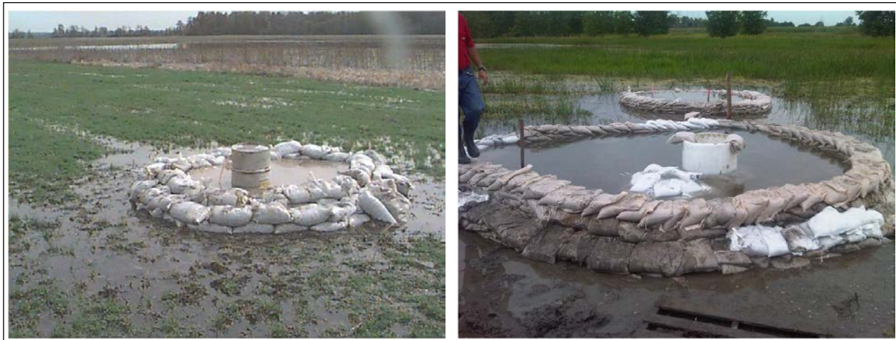
Figure K-14. Multiple Sand Bag Rings Built Around Ineffective Initial Barrel Control.
