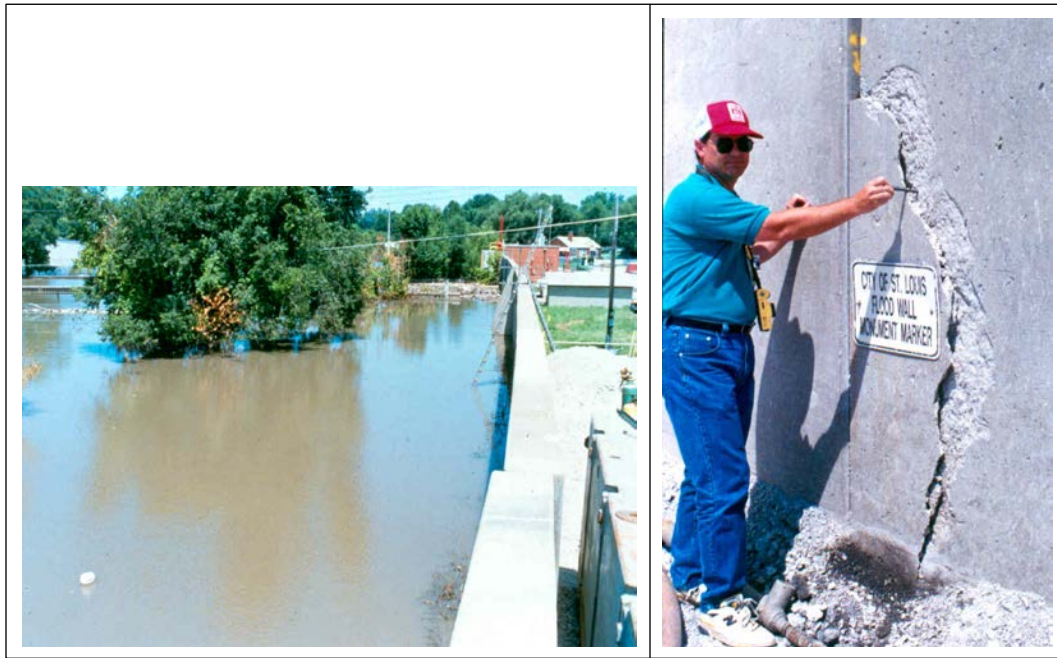
Figure K-10. Floodwall Differential Movement and Concrete Damage on Stem.
